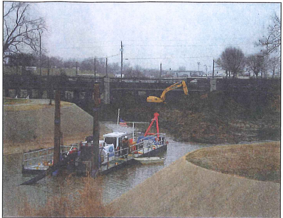
The dredge "Liberty" moves up the creek to remove a large stockpile of material that was pushed "down the creek" with dozers.
