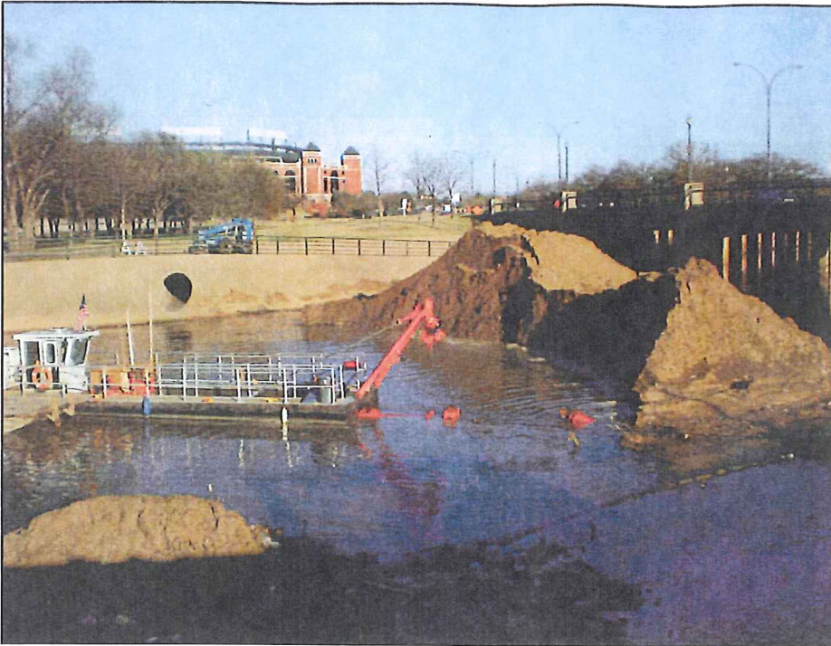
With Ranger Stadium in the background, the dredge chips away at the stockpiled material in the creek and pumps it 1.5 miles to a settling basin.
