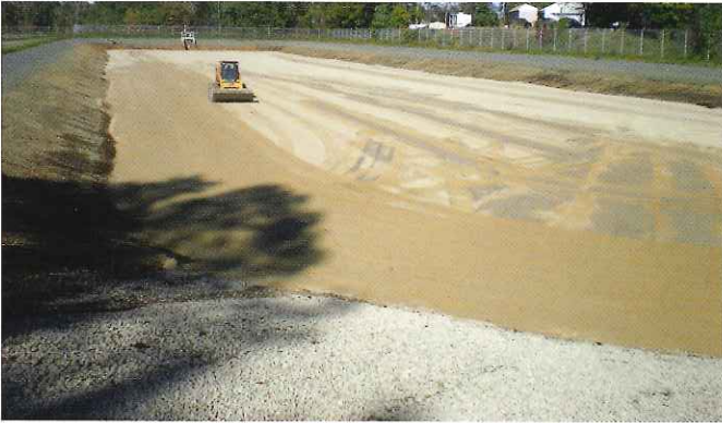
The final grading for reestablishing a settling lagoon.
