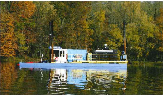
Hydraulic dredge in operation during a lake restoration project.
