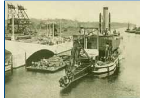
Ellicott 20" Dredge at work in Panama Canal Lock in 1913
