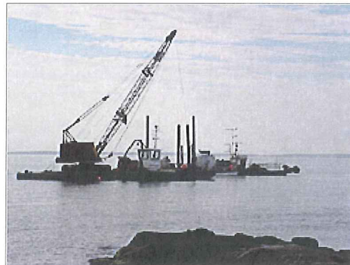
The County dredge at work.
