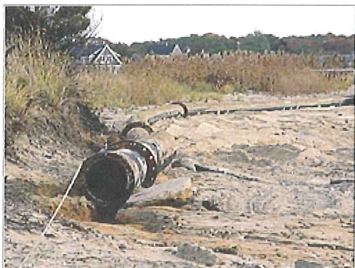
The 16" discharge tubes used in the process.
