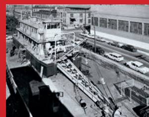
The Salina Cruz , completely assembled in a Baltimore, Maryland shipping yard, ready to be dismantled and loaded for a railway journey to Mexico - 1957
