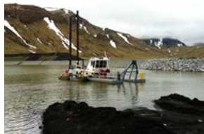
New fishing harbor being built with the help of an 1170 Dredge - Alaska, USA
