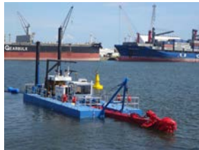
Port dredging with a 670 Dragon® Dredge - Guatemala
