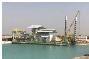
Custom B1190 Electric Wheel Dragon™ dredging hard material with Ellicott's patented Dual Wheel Excavator - Saudi Arabia
